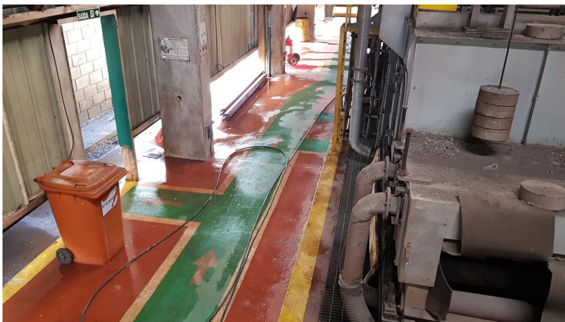
Limpeza geral – Shotblasting
