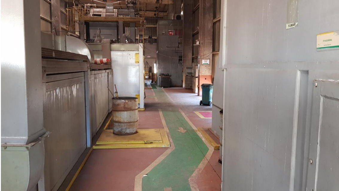
Limpeza geral – Shotblasting
