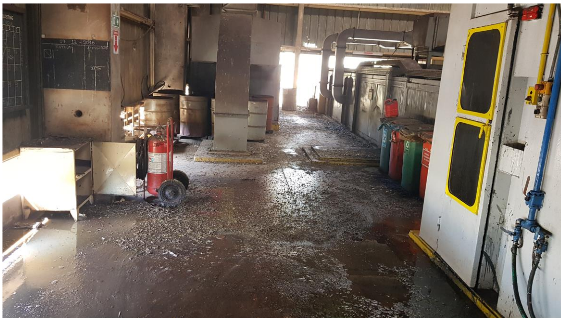
Limpeza geral – Shotblasting
